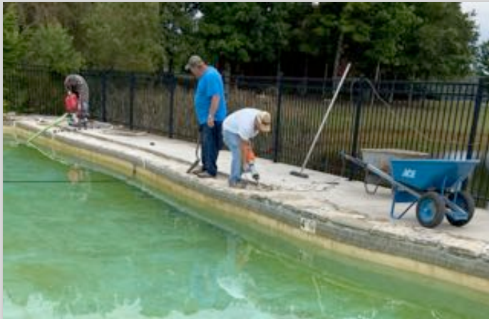
The rough tile around the edge of the pool has been removed and replaced with a smooth finish
